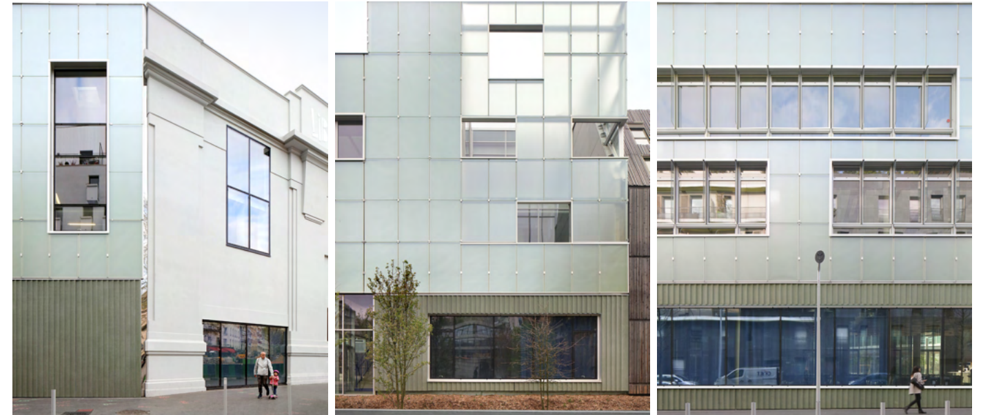
Detail of the junction between the historic pediment and the new façade, featuring a polished mirror joint.
